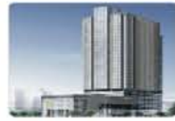
Nanjing Liao Building (388 households)
